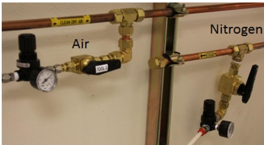
Figure 4: Rofin process Air and Nitrogen on/off valves.
