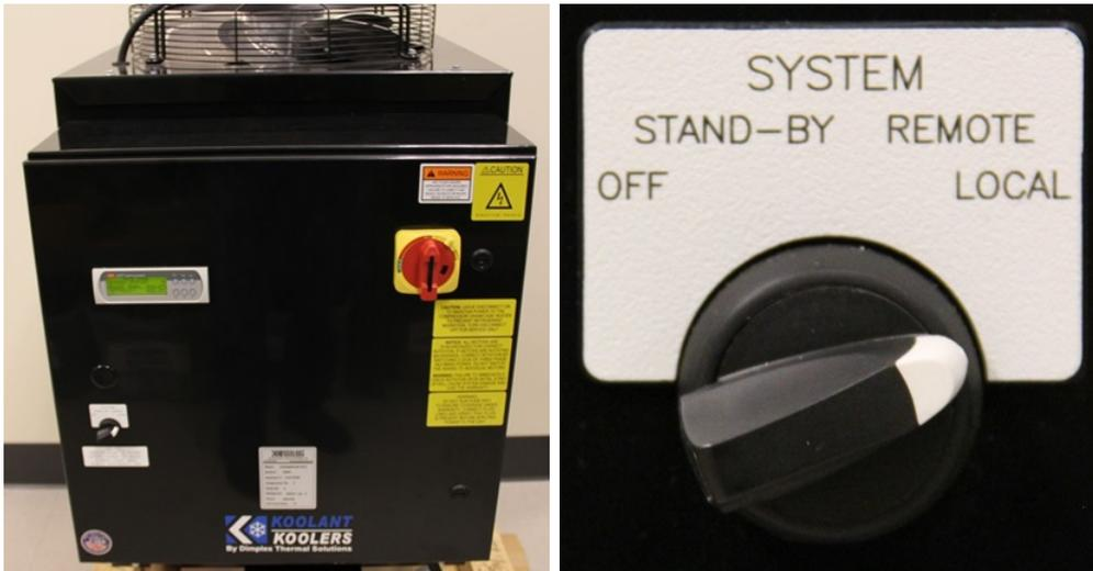
Figure 3: Rofin system chiller (left) and control switch (right).
